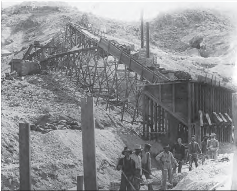
Above, The Bartlett #1 shaft with head frame, ore chute system, and storage bunker, at the town of Borate, Calico Mountains, pre-1897. White concentrate sits on a storage platform in the lower right of the photograph. F. M. "Borax" Smith's house is on the horizon, atop the hill. Smitheram collection.
