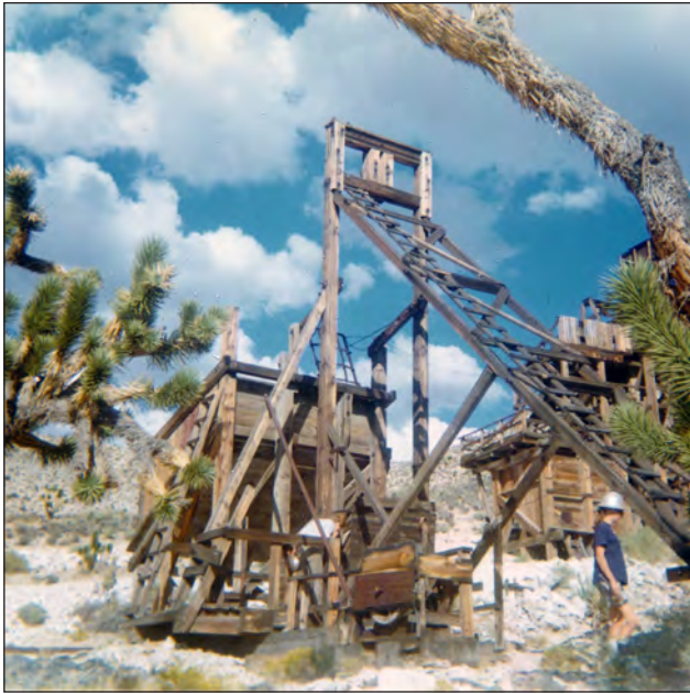
Evening Star mine, south headframe, 1967.
