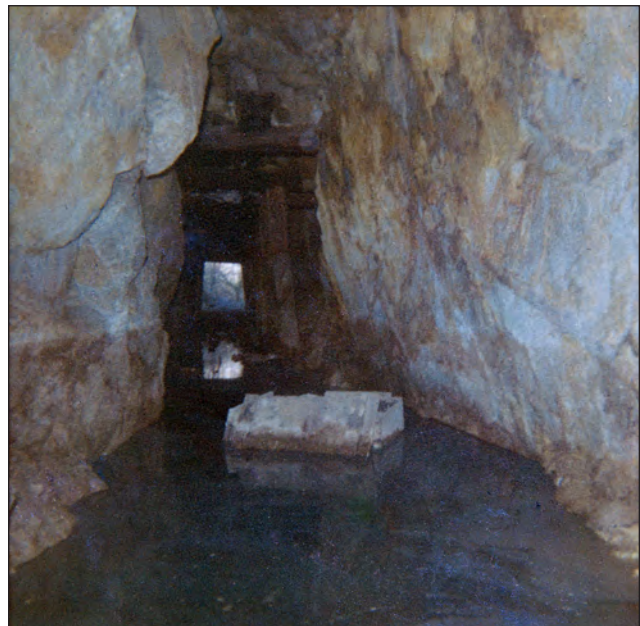
Flooded adit, view north toward entrance. Scanlon Gulch, 1966.
