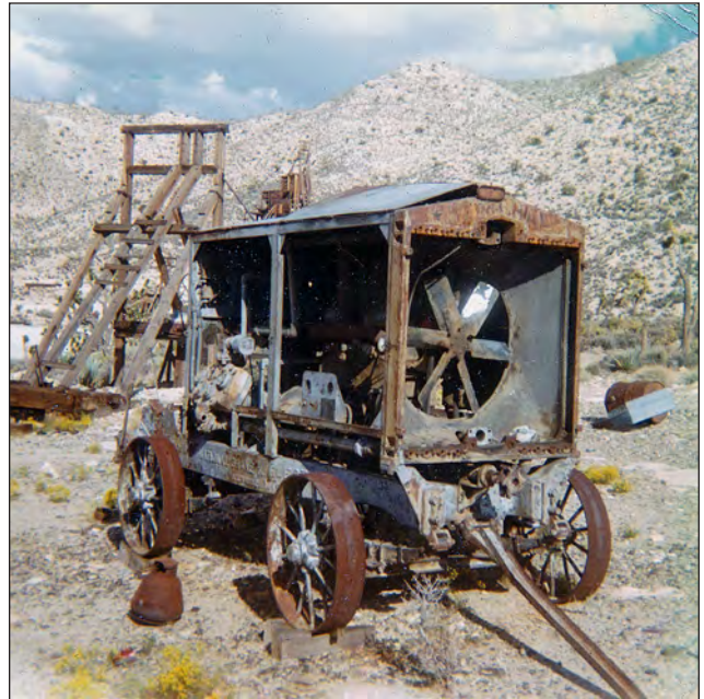
Evening Star mine, generator, 1967.
