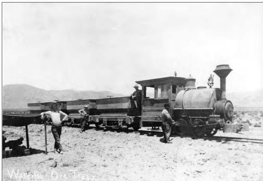
Figure 31. Waterloo Mine Railroad. O.A. Russell collection.
