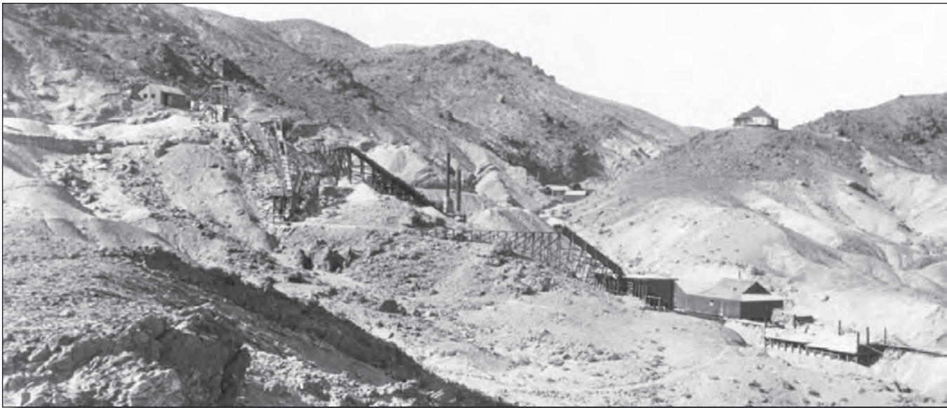
Above, The Bartlett #1 shaft with head frame, ore chute system, and storage bunker, at the town of Borate, Calico Mountains, pre-1897. White concentrate sits on a storage platform in the lower right of the photograph. F. M. "Borax" Smith's house is on the horizon, atop the hill. Smitheram collection.
