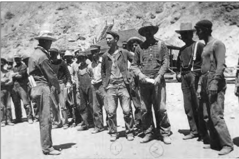
Figure 6. Mine workers and the shift boss at the town of Borate in front of the recreation room, after 1898. The Ella Pitchess house is top left; the Smith house peeks over the horizon. Wm. H. Smitheram collection
