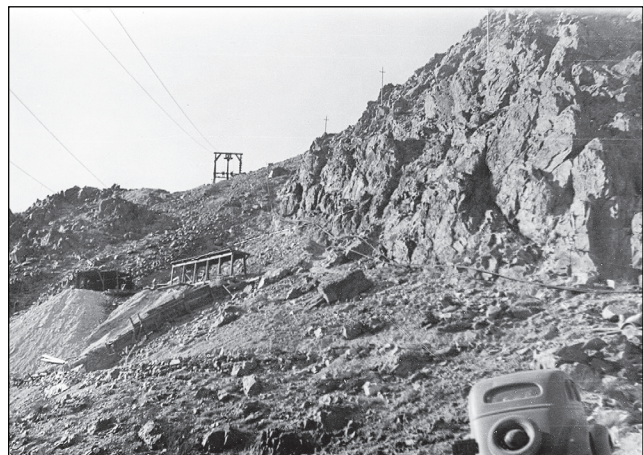
Fig. 11. Carlyle mill and lower mine workings, waste rock dump, aerial tram cables, and aerial tram tower on the skyline, ca. 1937. (NPS photo).
