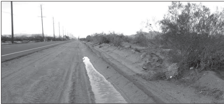
Figure 2. Standing water in a ditch near Lake Los Angeles following rain. Creosote is growing vigorously on the elevated ridge constructed when the road was built.
