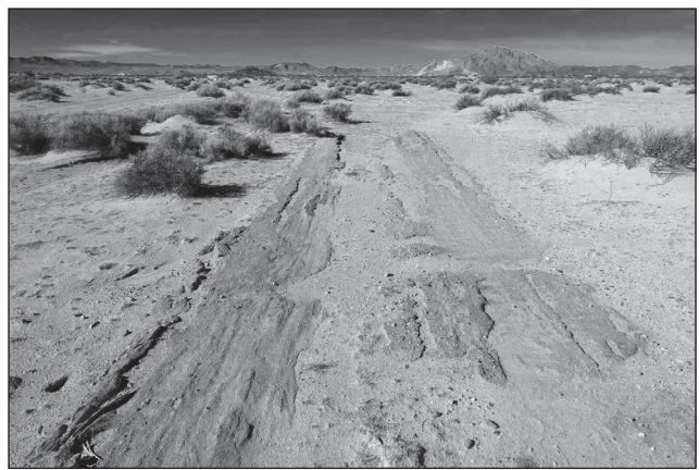
Figure 1-5. Telegraph road between Crucero and Mesquite Spring, stabilized with desert mix asphalt.
