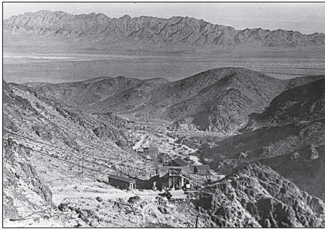
Fig. 8. Carlyle mill, ca.1937. Note aerial tram cables for transporting ore to the mill. ca. 1937 (NPS photo).
