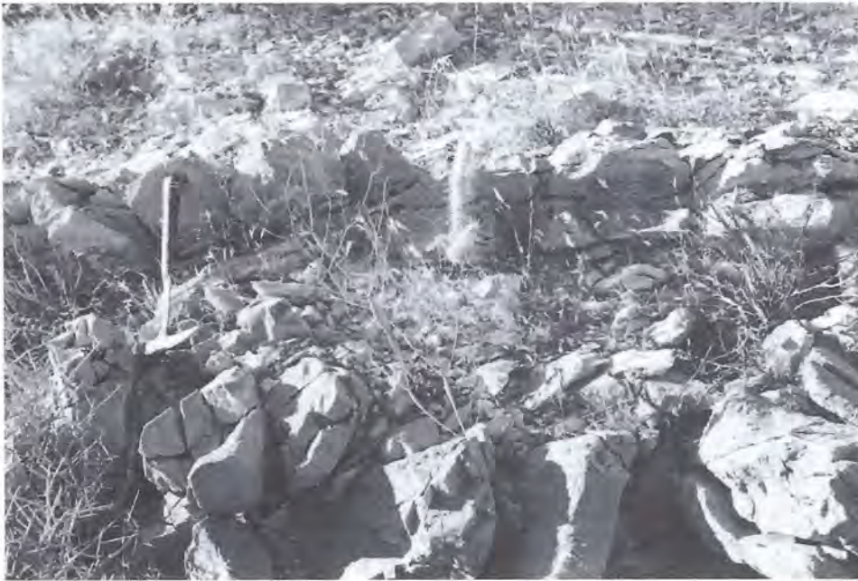
Figure 4. Footwall marble and juxtaposed hanging wall mylonitic Bonanza King. Plane of the fault lies just above the hammer head.
