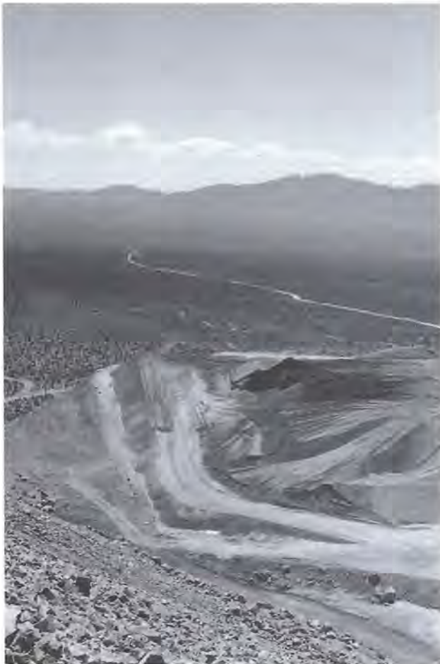
Figure 4. Morning Star leach pad, showing the buffer of sterile rock to guard against slumping or slipping of the crushed ore laden with cyanide solution. Photograph courtesy Bureau of Land Management.
