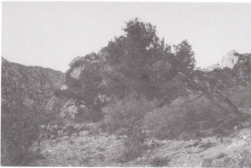
Figure 3. Rock foundations near the Giant Ledge mine. R.E. Reynolds photograph.
